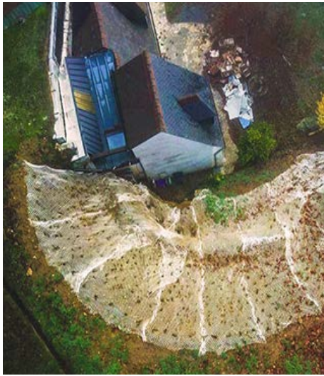
LITE-NET to support initial vegetation (picture taken from above)
